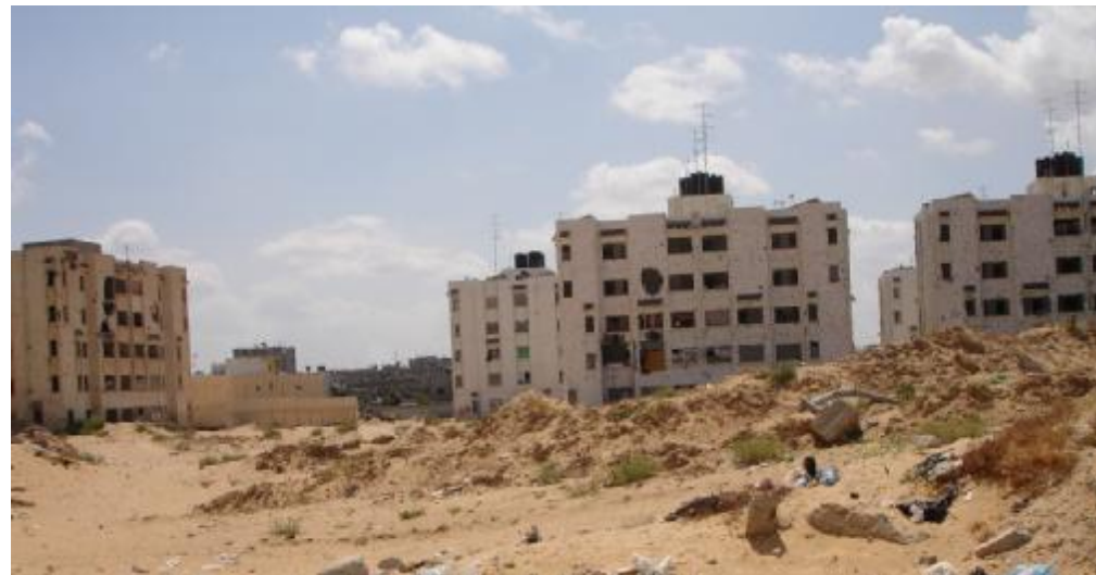
Figure S-8: EL-Farra project – nearby the AHP (damaged also)
