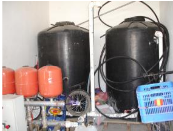
Figure C1-3: Water storage roof tanks and ground tanks with pumps
