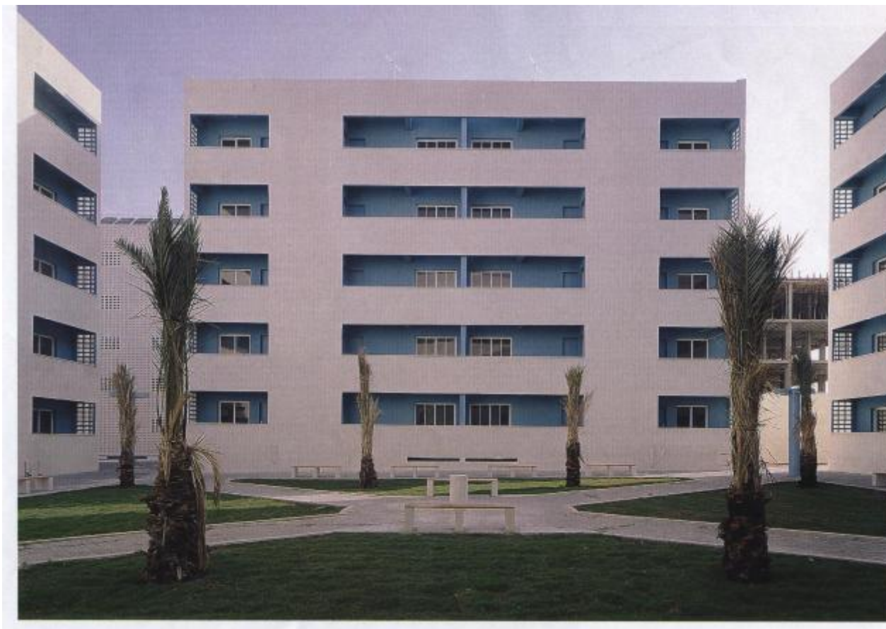
Figure C6-3: Photo of courtyards No. 1, No. 2 and No.3
