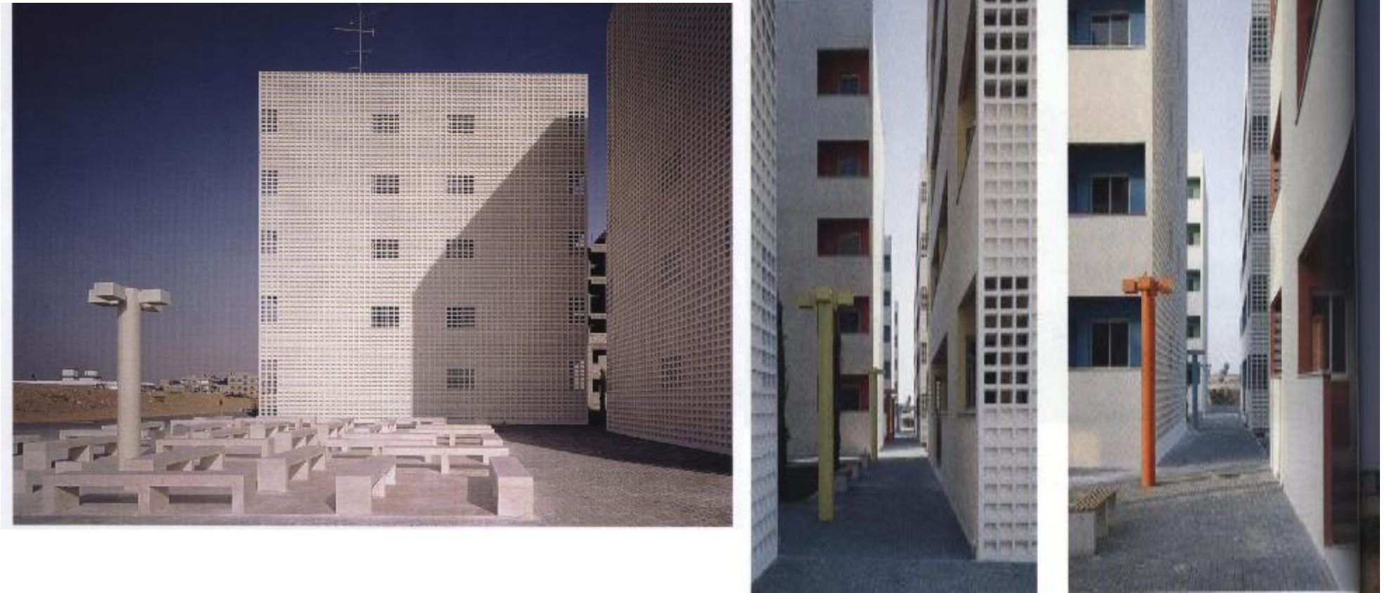
Figure C4-7: Security lighting - Cluster special Lighting poles
