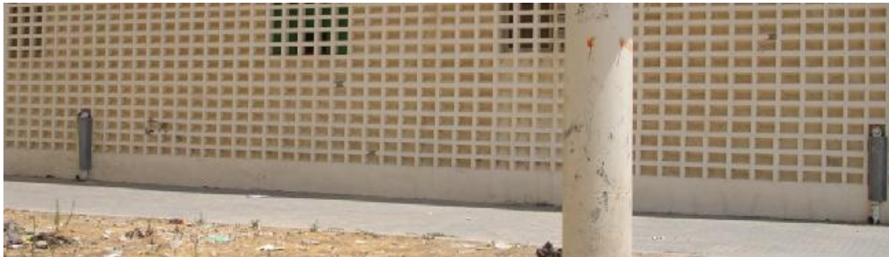
Figure C6-13: Roof drainage spouts opened into the footpaths
